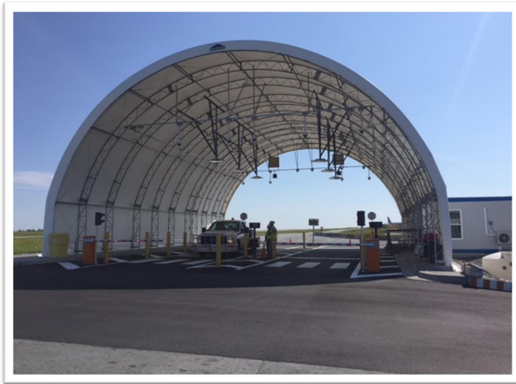
View of the exit from NPSV prior to entering the Critical Area
